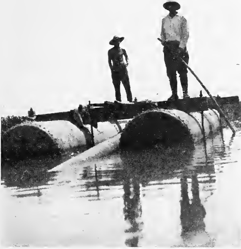
FLOATING THE PIPE LINE ACROSS THE RIVER
